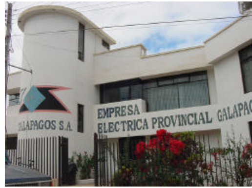
Fig.2: Main facade of the EGPG building
