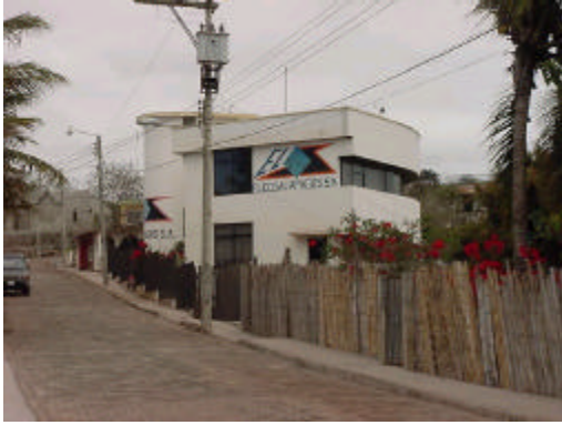
Fig.1: The EGPG building is located in Avenida Española
