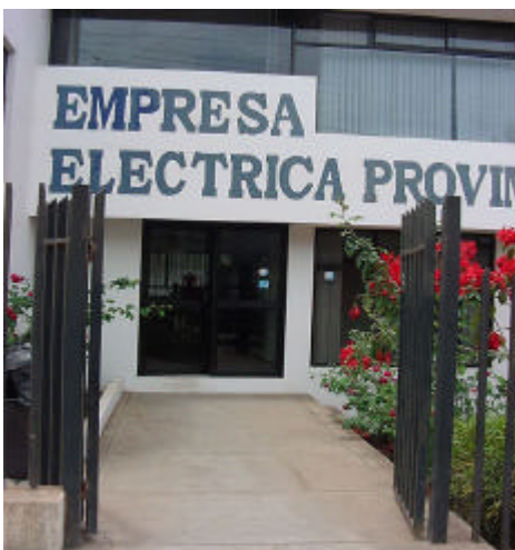
Fig.5: Glazed door of the main entrance
