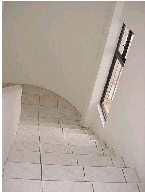
Fig. 8: Staircase with side windows
