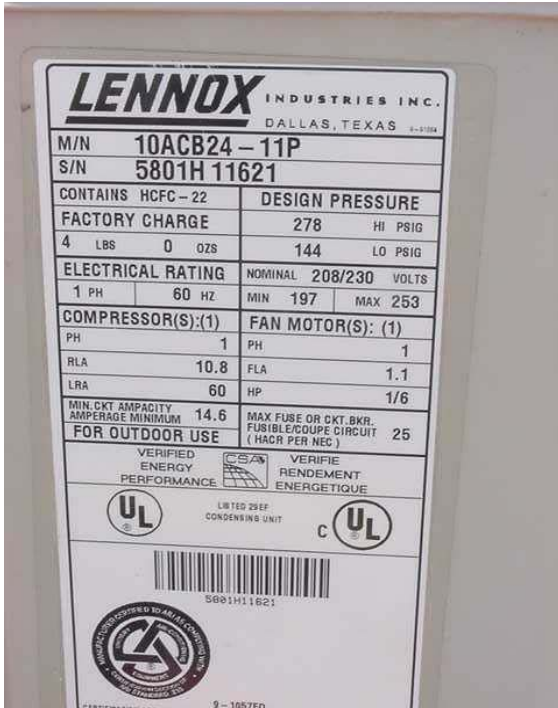
Fig. 21: Technical specifications of the Lennox A.C Fig.22: Tube fluorescent lamps inside diffusing glass ceiling bowl
