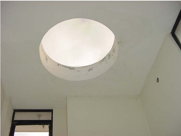
Fig. 12 : Glazed dome and side windows in the top of the staircase
