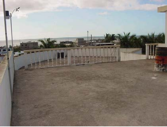
Fig. 11: Terrace on the roof of the building
