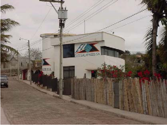
Fig.1: The EPGC building is located in Avenida Española
